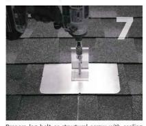
can no longer easily rotate. **DO NOT over-torque.** sure top of L-Foot makes solid contact with racking. NOTE: Structural screw can be driven with T-30 hex head bit.
