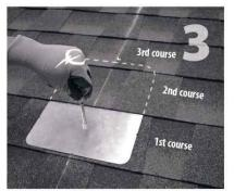
Locate, choose, and mark centers of rafters to be Carefully lift composition roof shingle with roofing Insert flashing between 1st and 2nd course. Slide Mark center for drilling.
