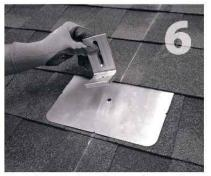
If attaching with lag bolt use a 1/32" bit (Lag). Use a Clean off any sawdust, and fill hole with sealant Place L-foot onto elevated flute and rotate L-foot to desired orientation.
