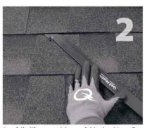
mounted. Select the courses of shingles where bar, just above placement of mount. Remove up so top edge of flashing is at least ¾" higher nails as required and backfill holes with aproved than the butt-edge of the 3rd course and lower sealant. See "Proper Flashing Placement" on next flashing edge is above the butt-edge of 1st course.
