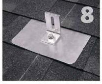
Prepare lag bolt or structural screw with sealing You are now ready for the rack of your choice. washer. Using a 1/2-inch socket on an impact gun, Follow all the directions of the rack manufacturer drive prepared lag bolt through L-foot until L-foot as well as the module manufacturer. NOTE: Make
