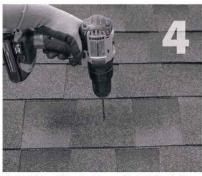
1/8" bit (ST) for attaching with the structural screw. compatible with roofing materials. Drill pilot hole into roof and rafter, taking care to drill square to the roof. Do not use mount as a drill guide. Drill a 2" deep hole into rafter
